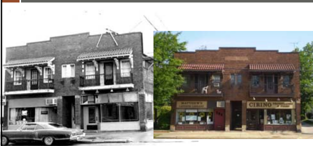
Built 1921 by contractor Charles A. Cahill, with a stepped parapet and tile-roofed balconies projecting from the upper level. Storefront transoms later covered and doors replaced among other modifications.
