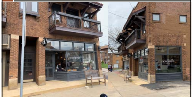
East storefront rehabilitated for Goodkind Coffee. Transom windows were uncovered and non-historic lighting removed with new signage installed.
