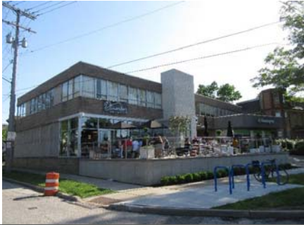
First floor converted to Dinerbar on Clifton restaurant, with compatible storefront replacement and new elevated outdoor dining terrace.
