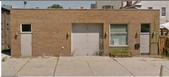
Before improvements: a non-descript one story warehouse building. Constructed 1924, façade alterations c.1990. (Lakewood Building Permit)
