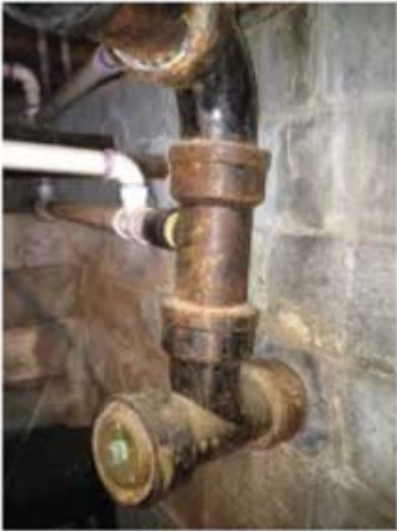
Typical Basement Thru Wall Sanitary Cleanout
