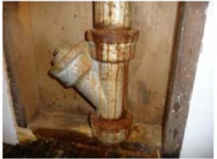
Typical Basement Floor Sanitary Cleanout
