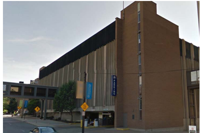
1422 Belle— South Parking Garage
